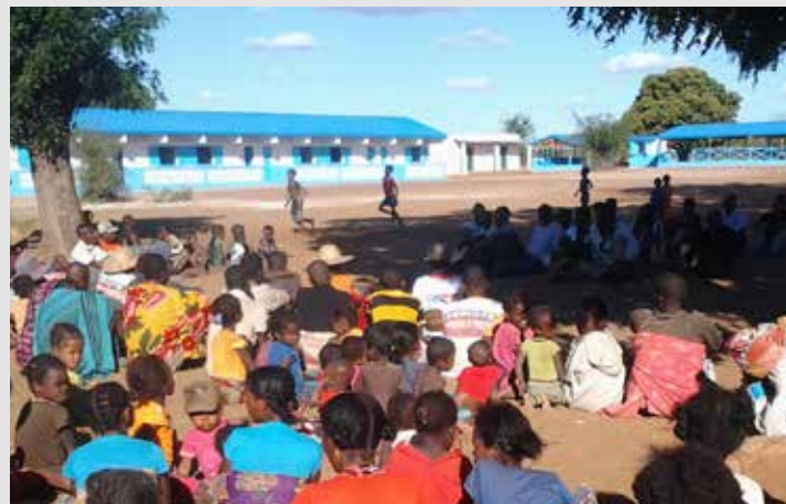
Two months to go and the school is already a huge attraction! From l-r: school, kitchen, canteen.
